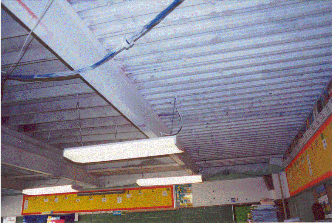
Figure 4: Classroom Building, interior of classroom
