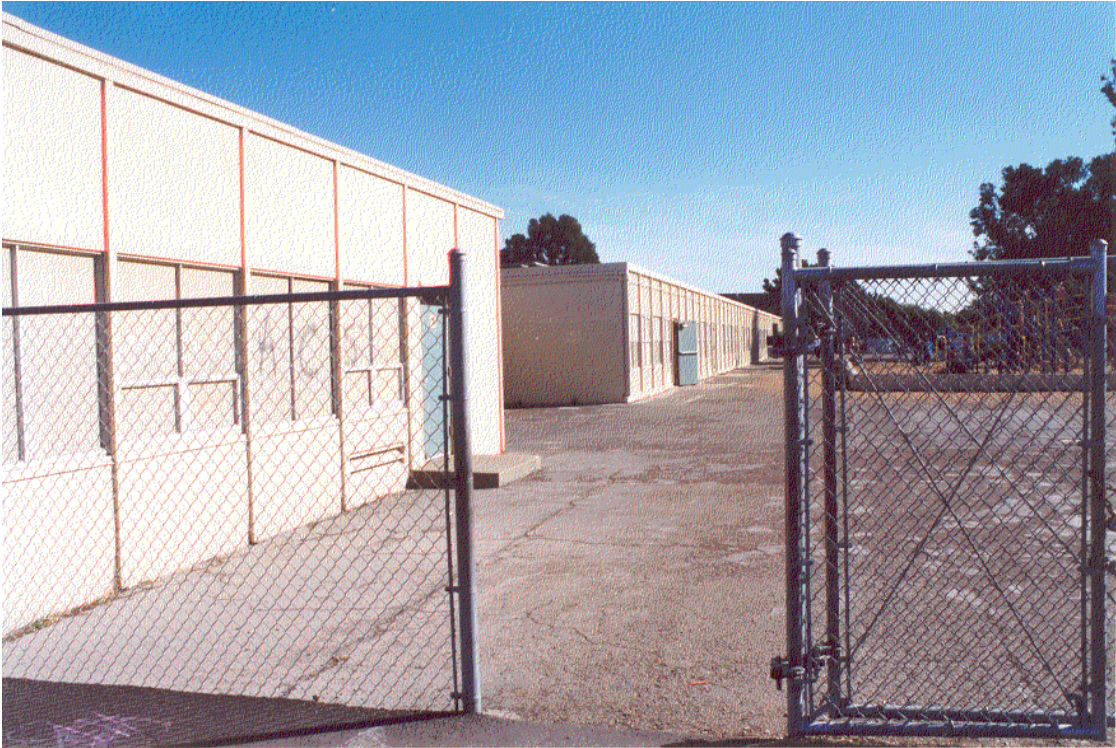
Figure 6: Classroom Building, south face
