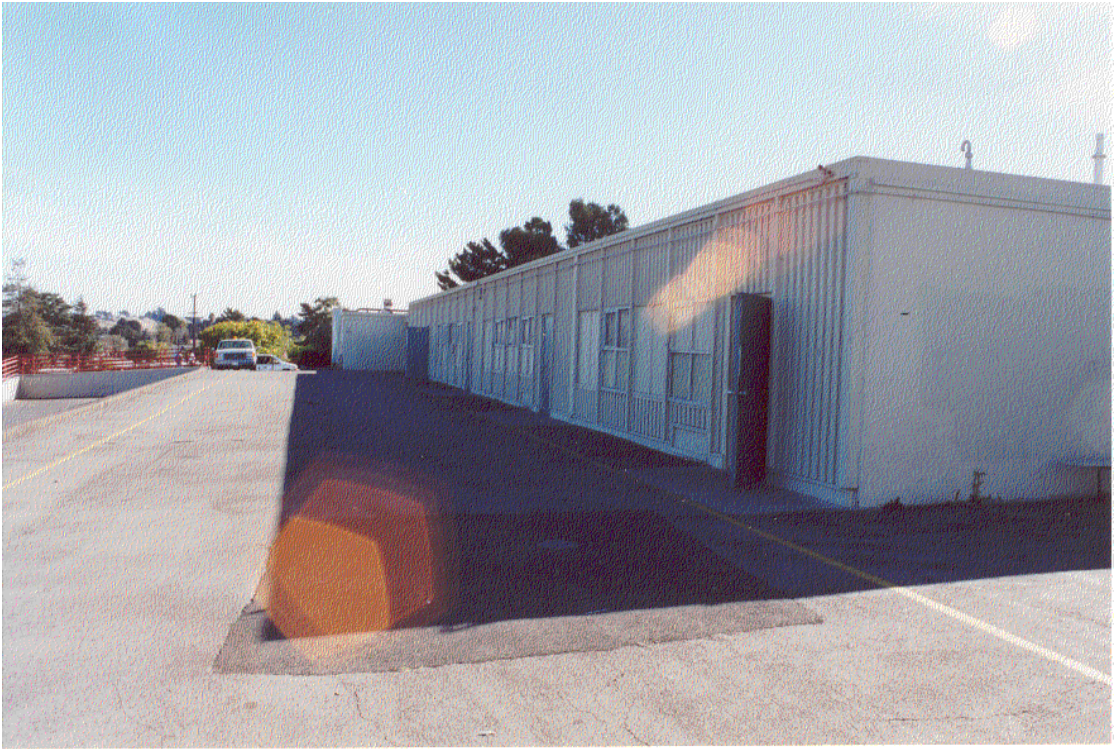
Figure 7: Classroom Building, north face
